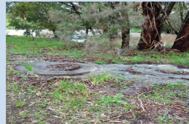
A sewer system surcharging from a manhole during peak weather event (>1 in 5 year event)
