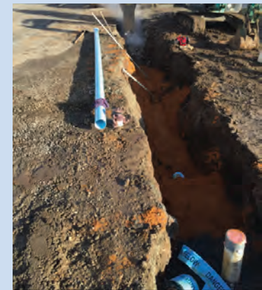
Trenching for a water main renewal project in Ballarat
