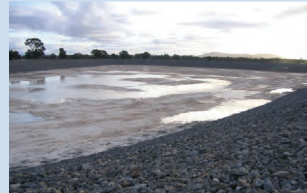
Construction of Maryborough's Bet Bet Storage Lagoon
