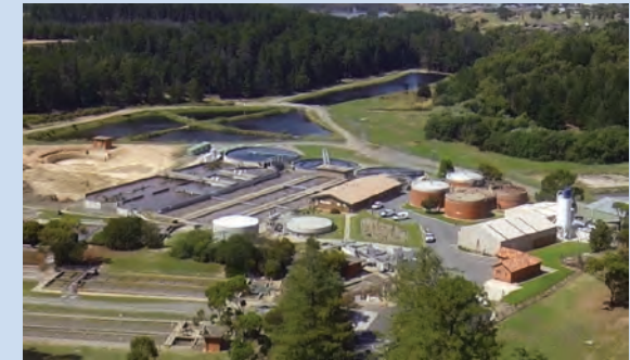
Overhead view of the Ballarat South WWTP
