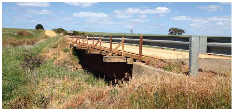
Bridge, photograph courtesy of Ararat Rural City Council.
