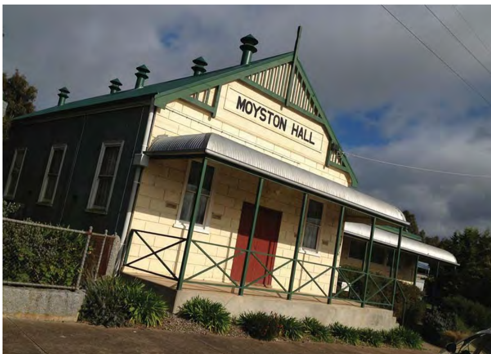
Moyston Hall, photograph courtesy of Ararat Rural City Council.
