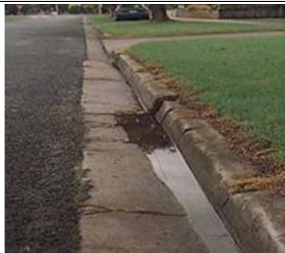
Figure 12: E amples of Kerb & Channel distress
