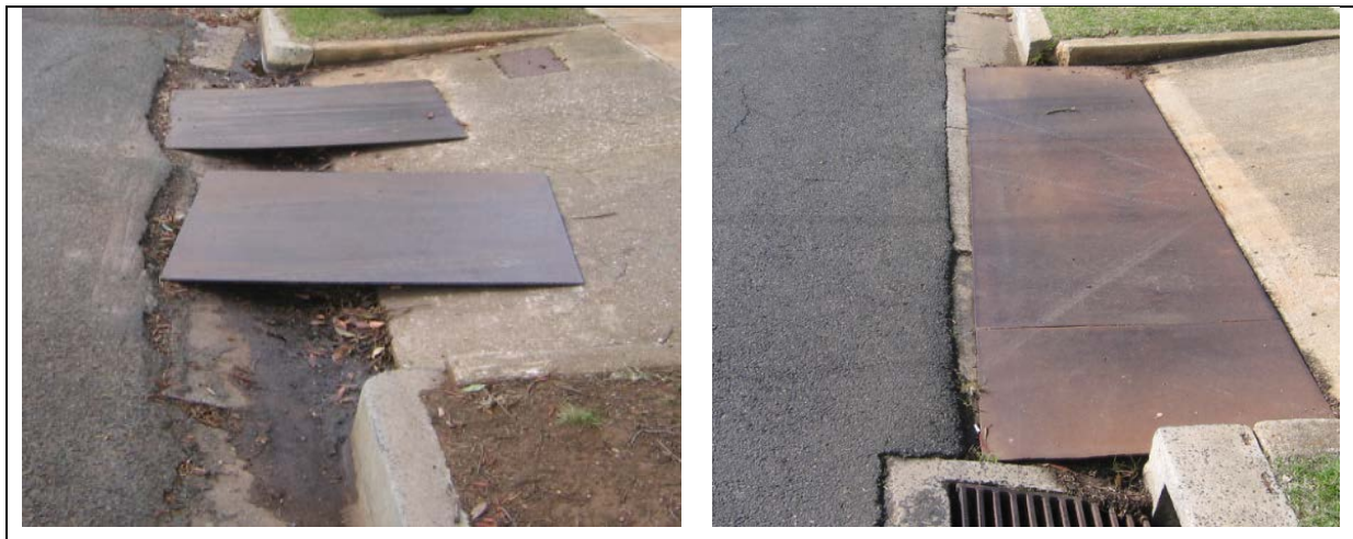
Figure 24: Problematic plated kerb ramps in Bacchus Marsh
