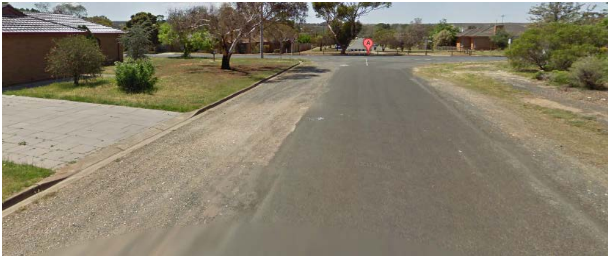
Figure 27: A bitumen strip down the centre of the road is no longer 'acceptable'
