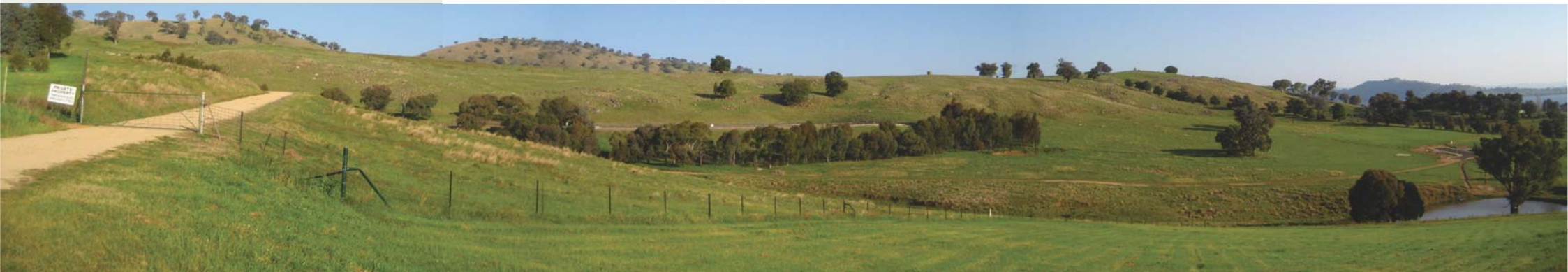
Sewerage Treatment Works
