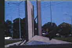
New central town entrance to clearly define town's street (Ottobius, Eastern Namibia, South Africa)
