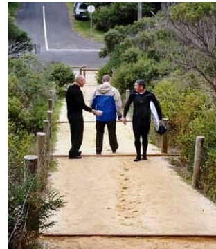
Steep path to Pt Lonsdale Back Beach subject to erosion
