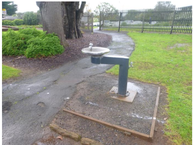
Existing drinking fountain near Entrance N°7
