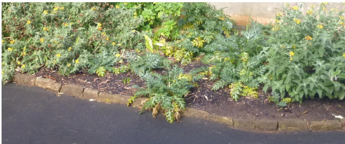
Existing limestone/sandstone soldier course edging at the edges to footpaths
