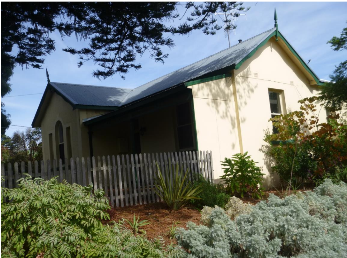
Existing Curator's Cottage
