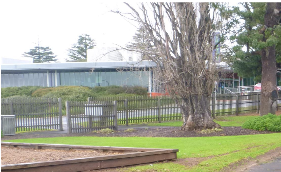
Existing conditions at Entrance N°7
